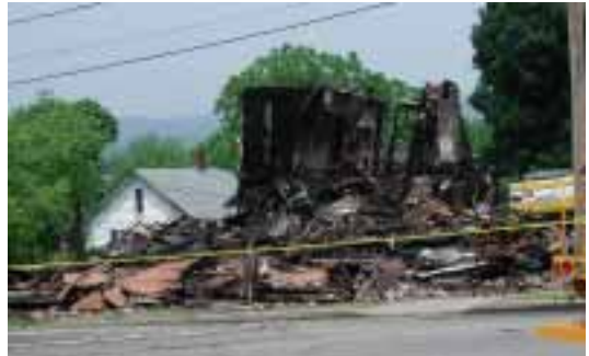
Above, the building that housed Rascals Brass Rail, after the June 11 fire.
